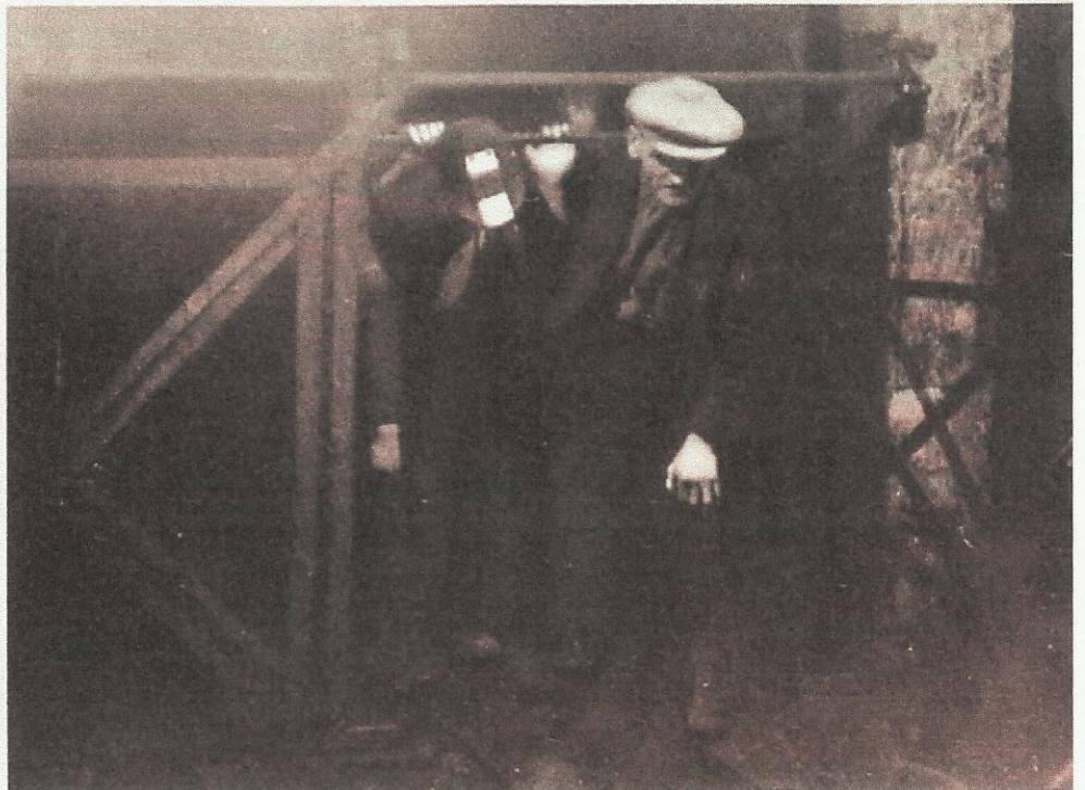
5 500 ft. Below Ground He Comes Out of the Cage The 500 ft. journey has taken them only a few seconds. Over 100 men are working on the night shift. As they leave the cage their places are taken by the stone-men, who have been blasting away the stone so that the miners can get at the coal.
